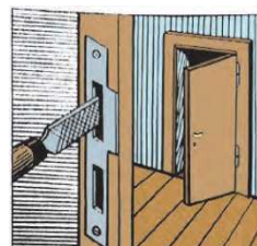
4-rasm. Uyalarni egovlab moslash.
