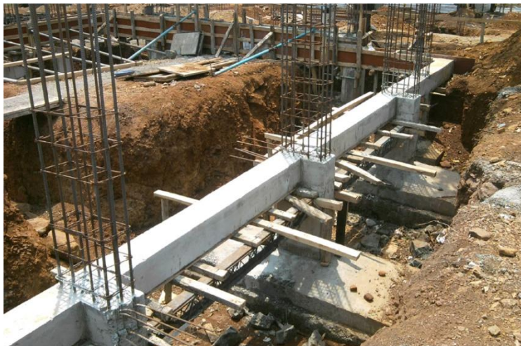
2-rasm. Tasma yordamida o‘zaro bog‘langan aloxida poydevorlar
