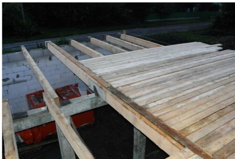
4-rasm. Yog'och to'sinli orayopma
