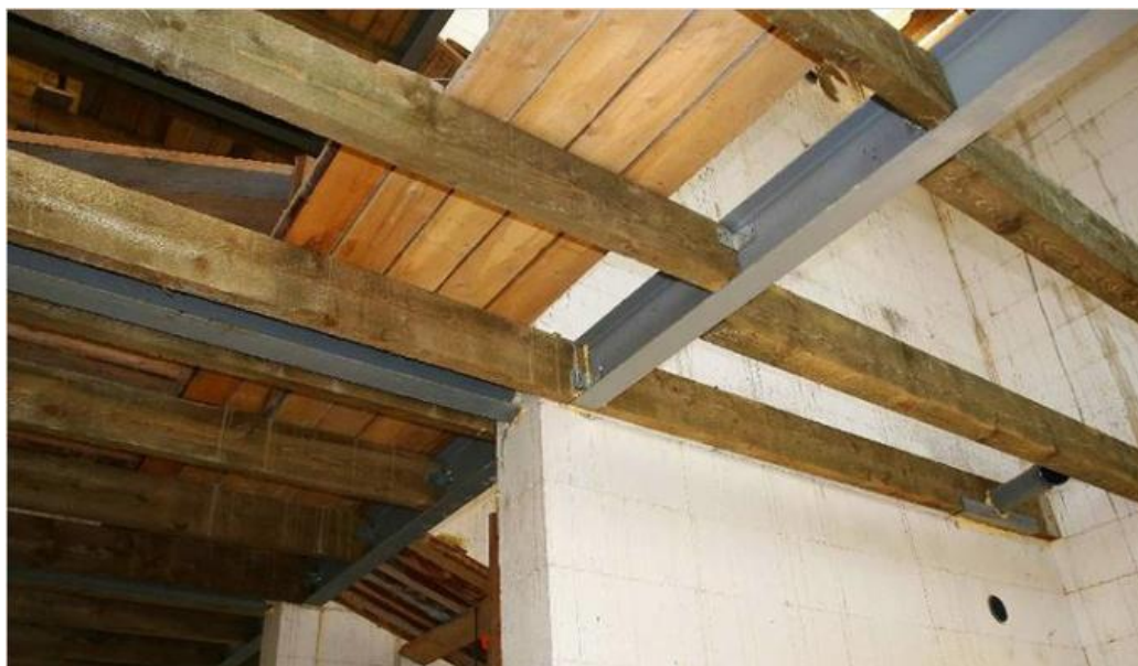
5-rasm. Yog'och va metal to'sinli orayopmalar
