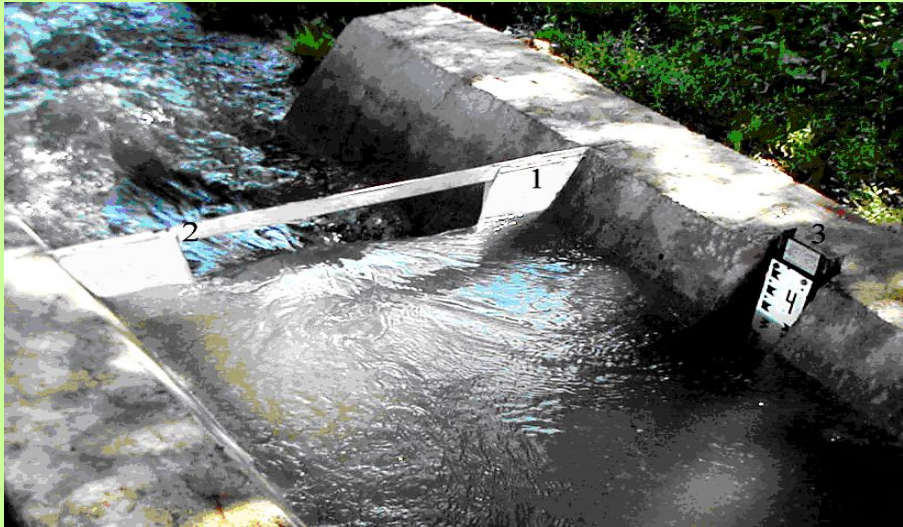
9-rasm. Chipoletti suv o'lchagichli gidropost.
