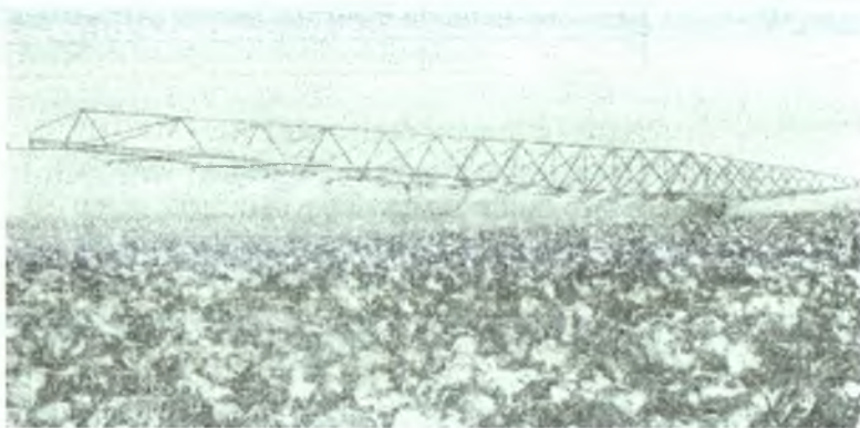
17-rasm. g'o'zani ikki qanotli yomg'irlatish (DDA-100M) mashinasi yordamida sug'orish.
