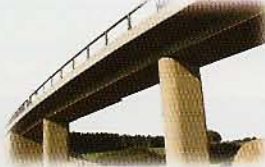
a concrete bridge
