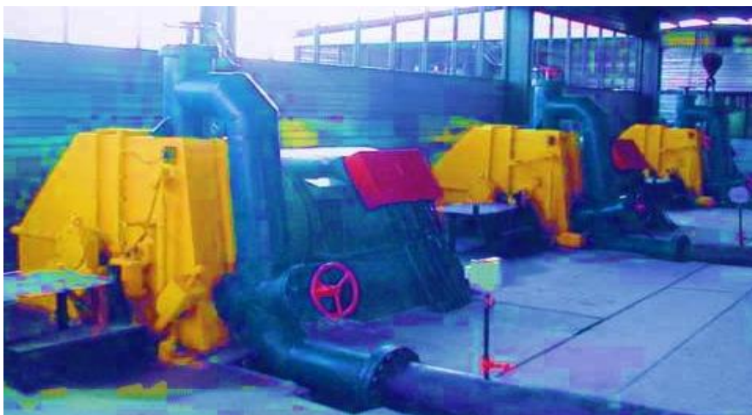
3.15-rasm. Vertikal o'rnatilgan cho'michli ish g'ildirakli kichik GES mashina zalining ko'rinishi
