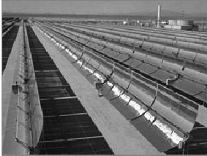
Figure 10.18 Concentrating solar collector of the parabolic trough type. (Image courtesy of the U.S. Department of Energy, Washington, DC, is in the public domain.)
