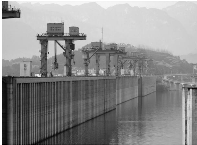
Figure 8.1 The Three Gorges Dam is the largest operating hydroelectric power stations at an installed capacity of 22,500 MW.
