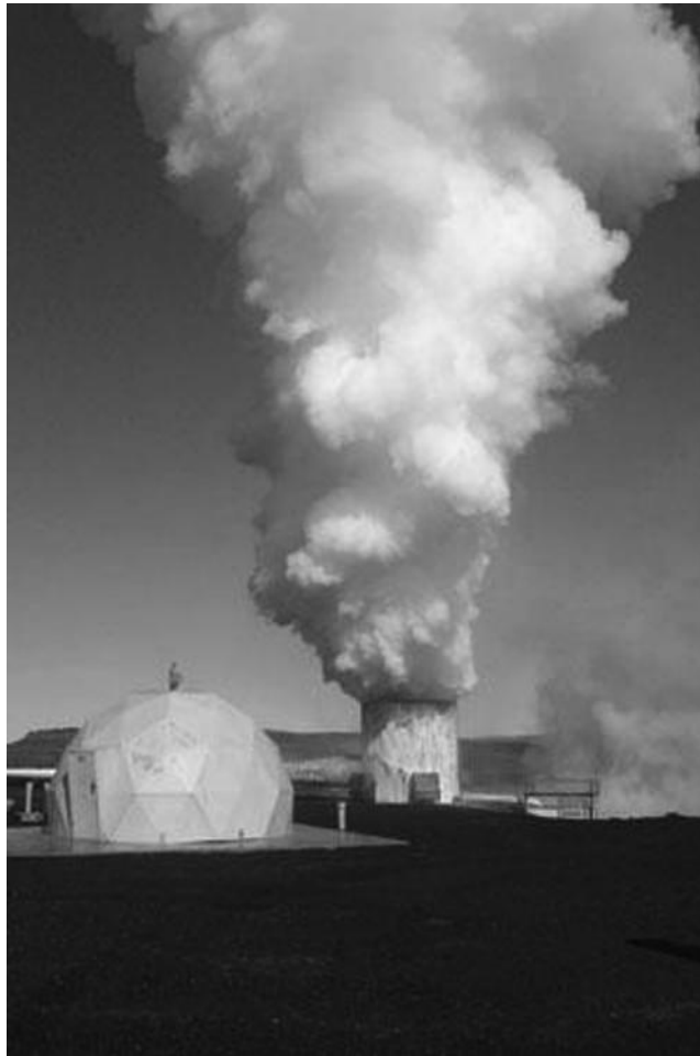
Figure 6.1 Geothermal borehole outside the Reykjavik Power Station. (Photo taken by Yomangani, and released to the public domain; http://en.wikipedia.org/wiki/Geothermal_power_in_Iceland )
