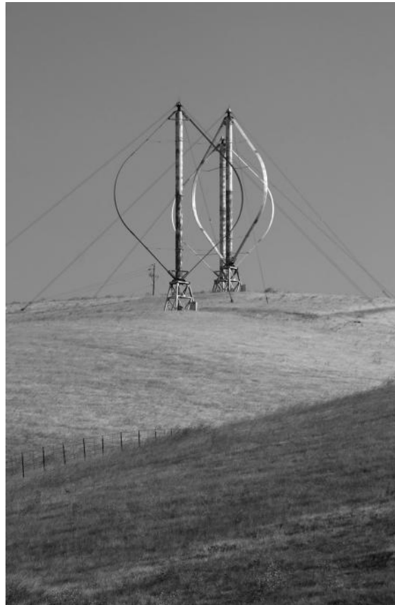
Figure 7.15 Example of a vertical axis turbine of the Darrieus design.
