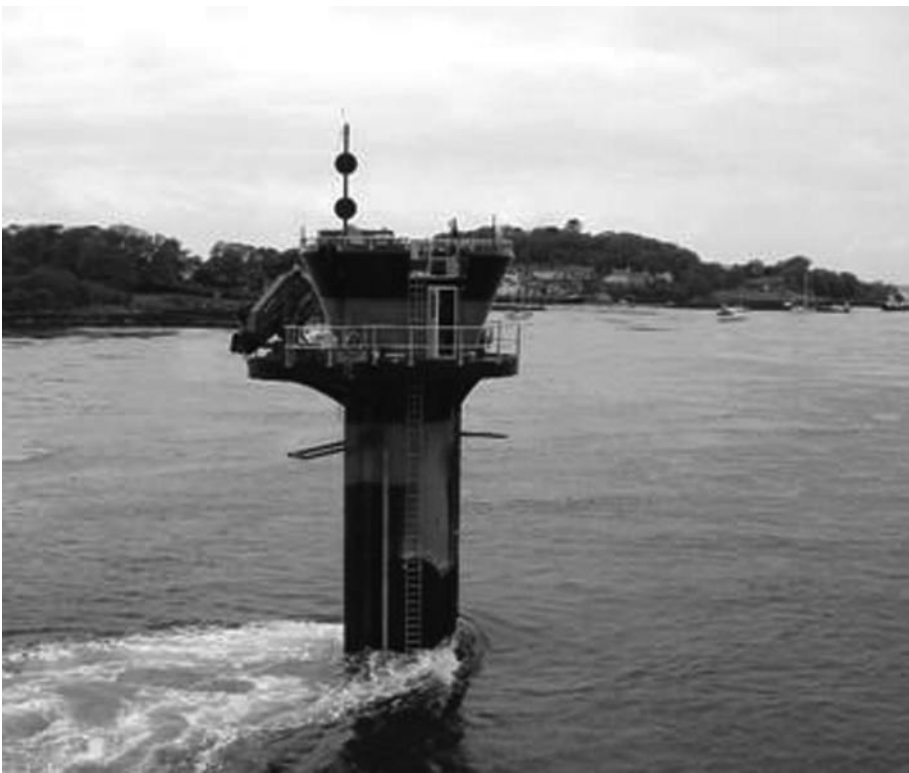
Figure 8.16 A commercial tidal current generator made by Seagen installed in Strangford Lough, Northern Ireland. The underwater tidal currents drive turbines. Note the visible wake indicating the current's strength. (Image by Fundy is licensed under the Creative Commons Attribution-Share Alike 3.0 Unported license, http://en.wikipedia.org/wiki/File:SeaGen_installed.jpg )
