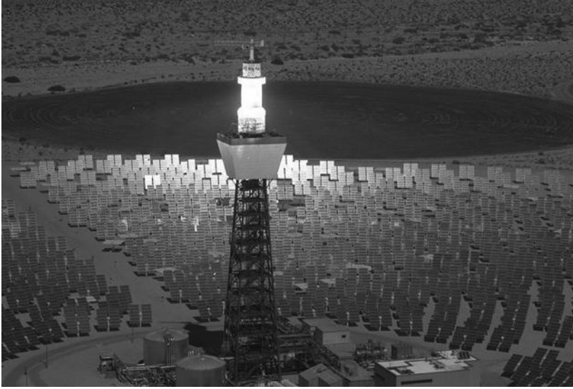
Figure 10.20 A power tower solar concentrator system. (Image courtesy of the U.S. Department of Energy, Washington, DC, is in the public domain.)
