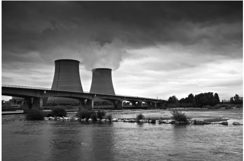
Figure 4.1 Nuclear power plant and the reactor cooling towers in France—a nation that leads the world in the percentage of its electricity generated by nuclear power at 78%. The large plumes emitted from the reactor cooling towers consist of water vapor.
