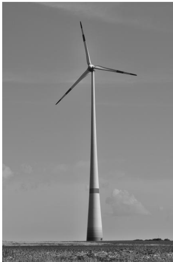
Figure 7.11 Although wind turbines rated at 10 MW are under development by several companies, the largest ones built to date by the German company Enercon have a rotor diameter of 126 m (413 ft) and a power rating of 7.58 MW.
