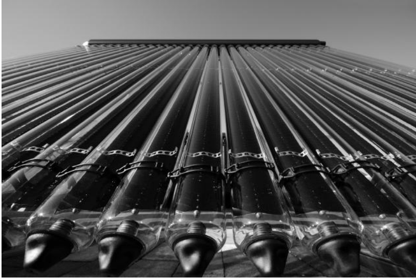
Figure 10.4 An evacuated tube solar water heater.
