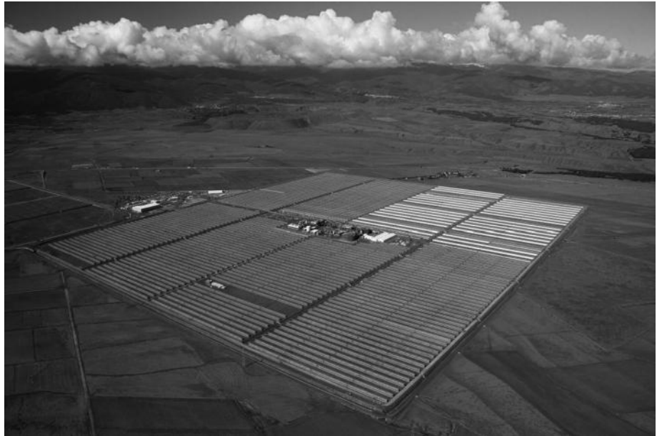
Figure 13.2 World's first commercial solar thermal power plant using molten salt storage built in Andalusia, Spain, in 2009. The long rows are parabolic mirrors that concentrate the solar energy onto tubes carrying molten salt to storage tanks in the middle of the picture. (Image by BSMPs is licensed under the Creative Commons Attribution-Share Alike 3.0 Unported, 2.5 Generic, 2.0 Generic, and 1.0 Generic license, http://en.wikipedia.org/wiki/File:12-05-08_AS1.JPG )
