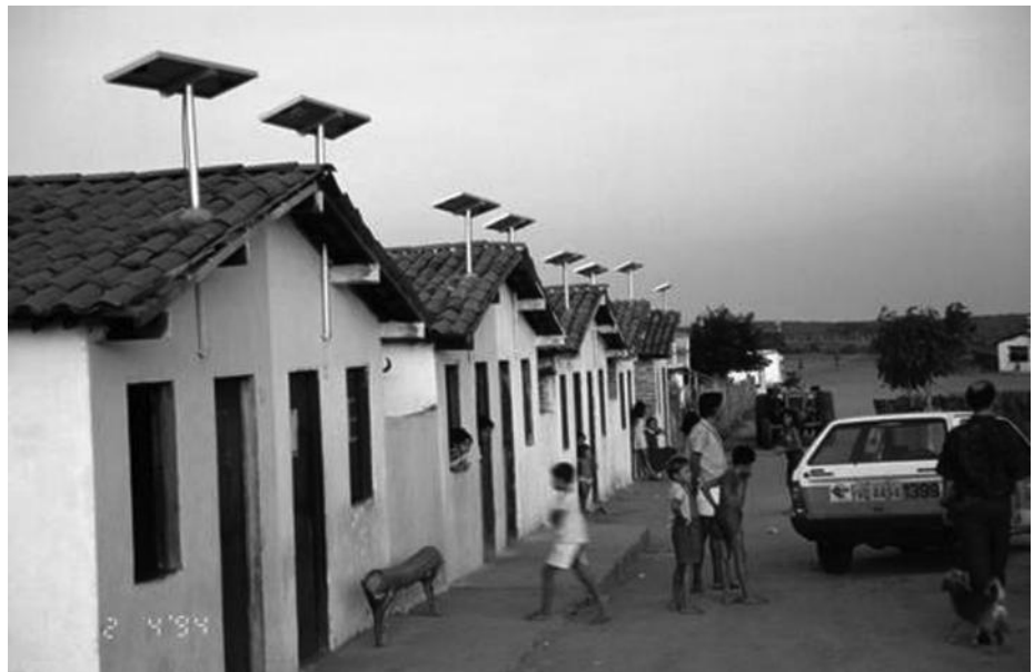
Figure 11.2 Fifty Watt solar panels on the roofs of a rural Columbian village. (Image courtesy of the U.S. Department of Energy, Washington, DC, is in the public domain.)
