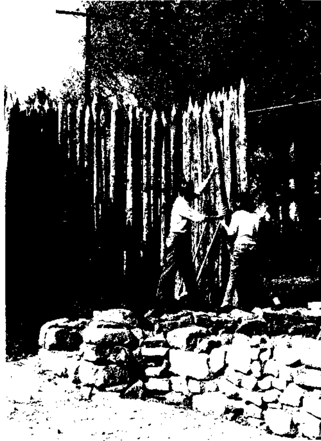
Placing palisade posts in the original Bethabara Tort Ditch.
