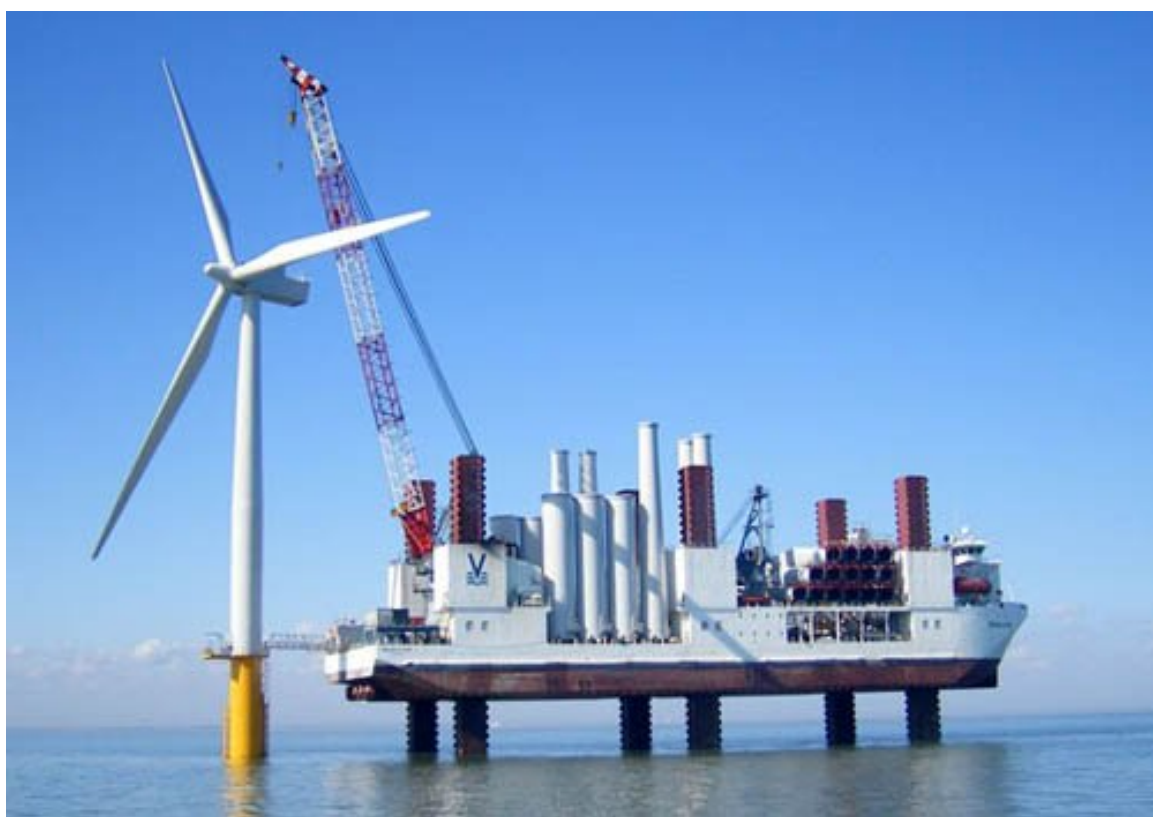
13-rasm. Eng katta quvvatli offshor shamol elektroqurilmalarini o‘rnatish.
