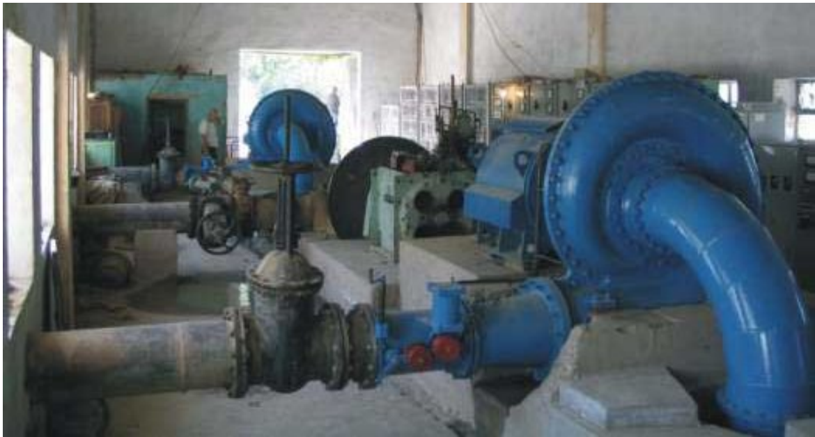
42-rasm. Gorizontial radial-o‘qiy turbinalar o‘rnatilgan kichik GES binosining ko‘rinishi.
